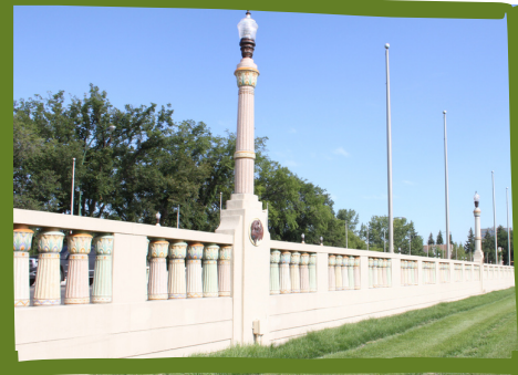
ALBERT STREET MEMORIAL BRIDGE
